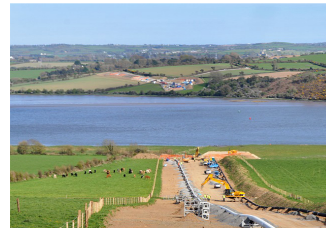
IMAGE 1.12 IMAGES SHOWING TYPICAL PIPELINE INSTALLATION AND CONSTRUCTION WORKING WIDTH AND ITS REINSTATEMENT
