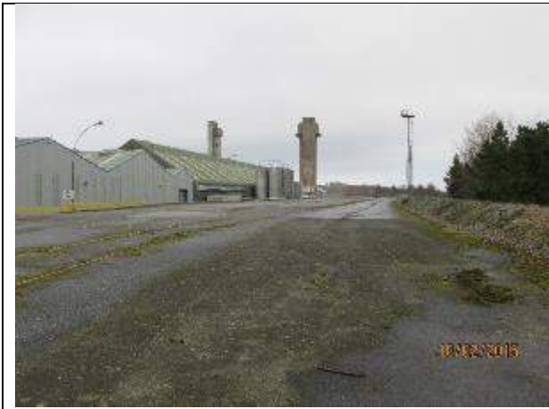
7. Site condition near IFI bridge
