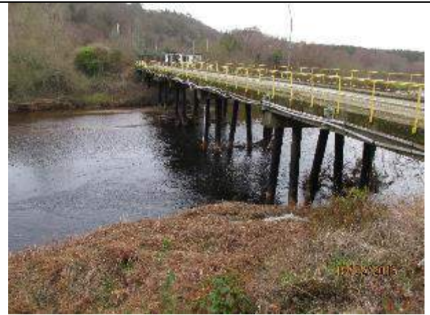
2. Downstream face of IFI bridge
