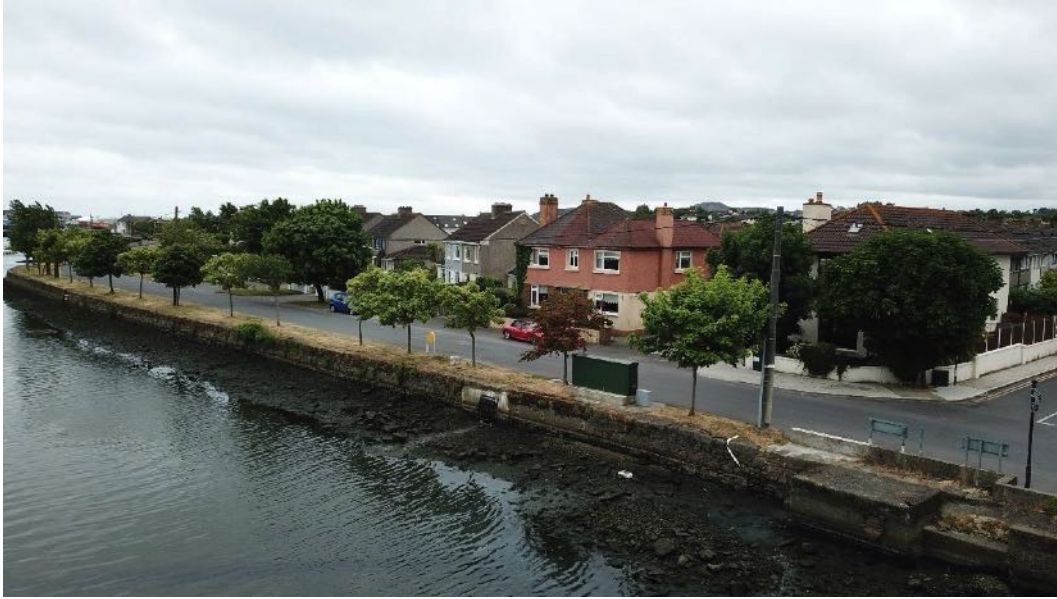
Figure 2.5: South Quay (viewed from the river channel)
