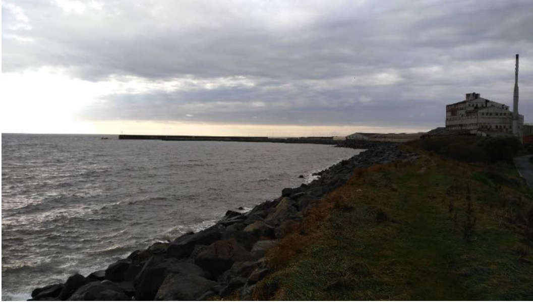
Figure 2.9: Irish Sea and existing revetment adjoining the Old Wallboard site (viewed from the existing revetment to the west of the site)
