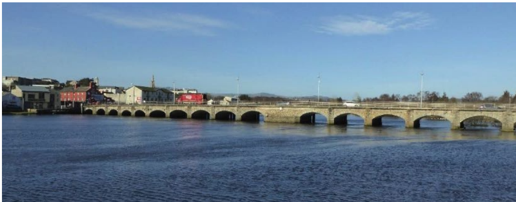
Figure 2.4: Arklow Bridge (viewed from downstream on North Quay)
