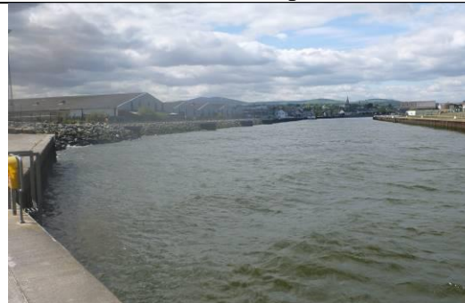
Plate 8: View upstream from breakwater
