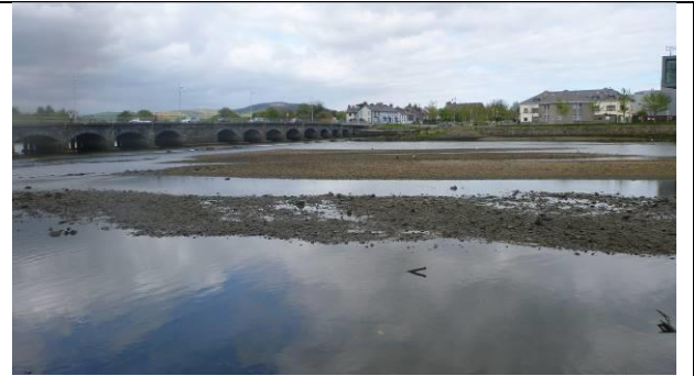
Plate 10: Gravel banks just downstream of bridge
