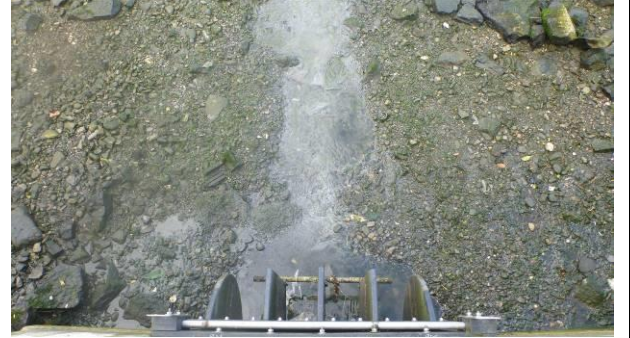
Plate 12: Sewage fungus at flap valve on the South Quay
