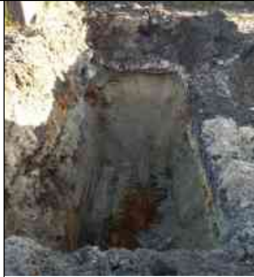
Photo 42: East-northeast view of TP4
