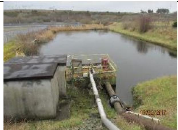
12. Attenuation pond at SE corner of plot A with pumped discharge arrangement
