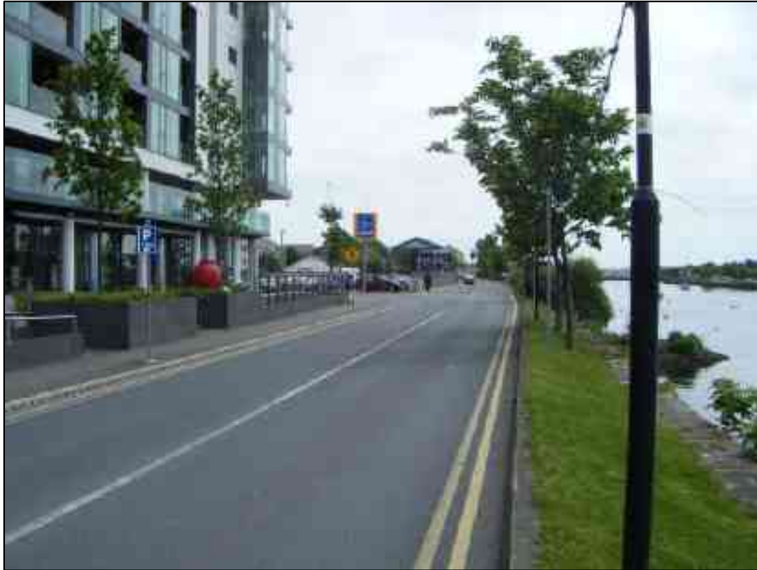
Figure 20 View of the west end of Section 4, looking southeast
