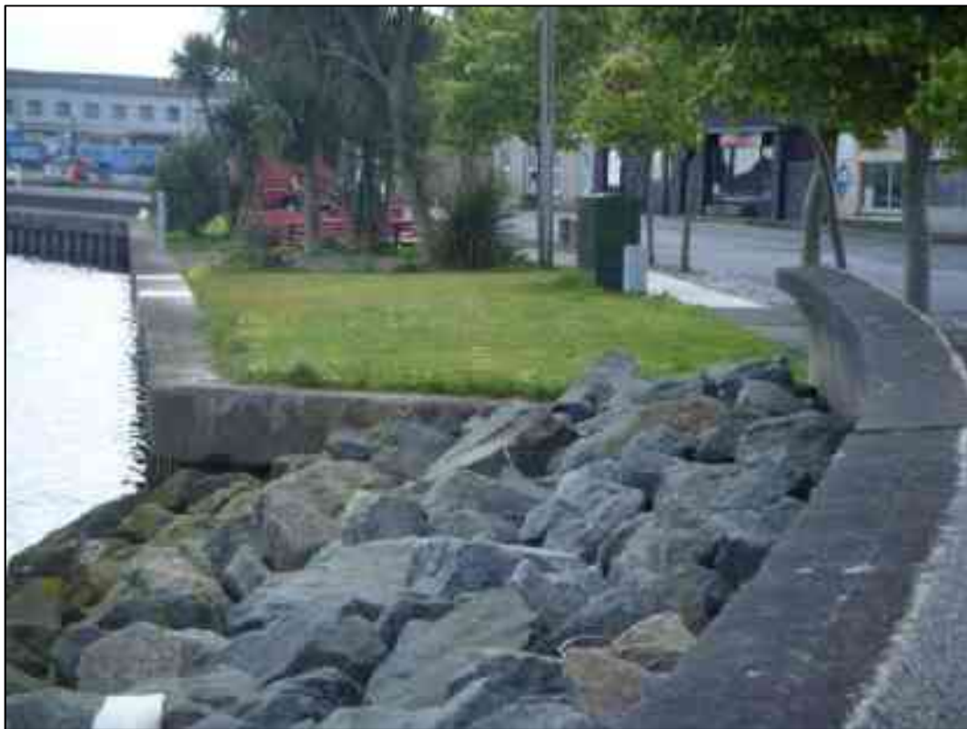
Figure 18 View showing return on sheet pile wall at the east end of Section 3
