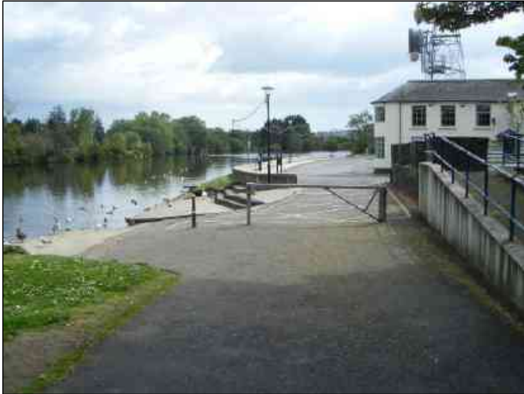
Figure 8 View of the intersection of the footpath and carriageway at the western end of Section 1
