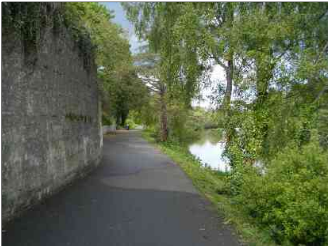
Figure 9 View of the footpath at the west end of Section 1 (note restriction caused by retaining wall)
