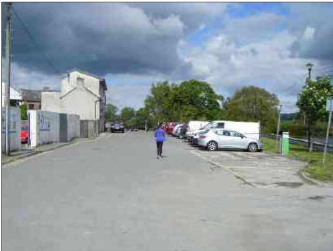
Figure 7 View of the carriageway in the eastern third of Section 1
