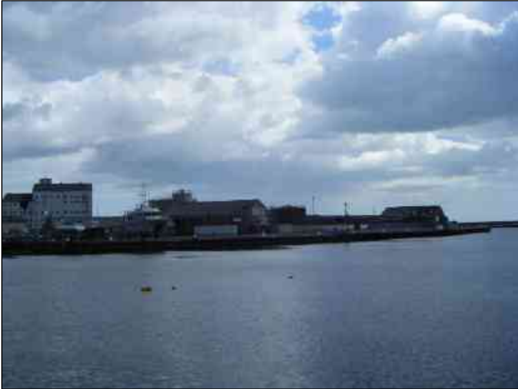
Figure 4 View of the proposed river crossing location, looking northeast.
