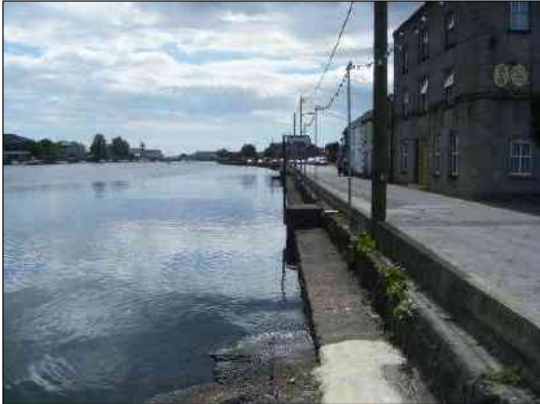
Figure 11 View of the existing stone wall along the South Quay (note encasement containing existing combined sewer)
