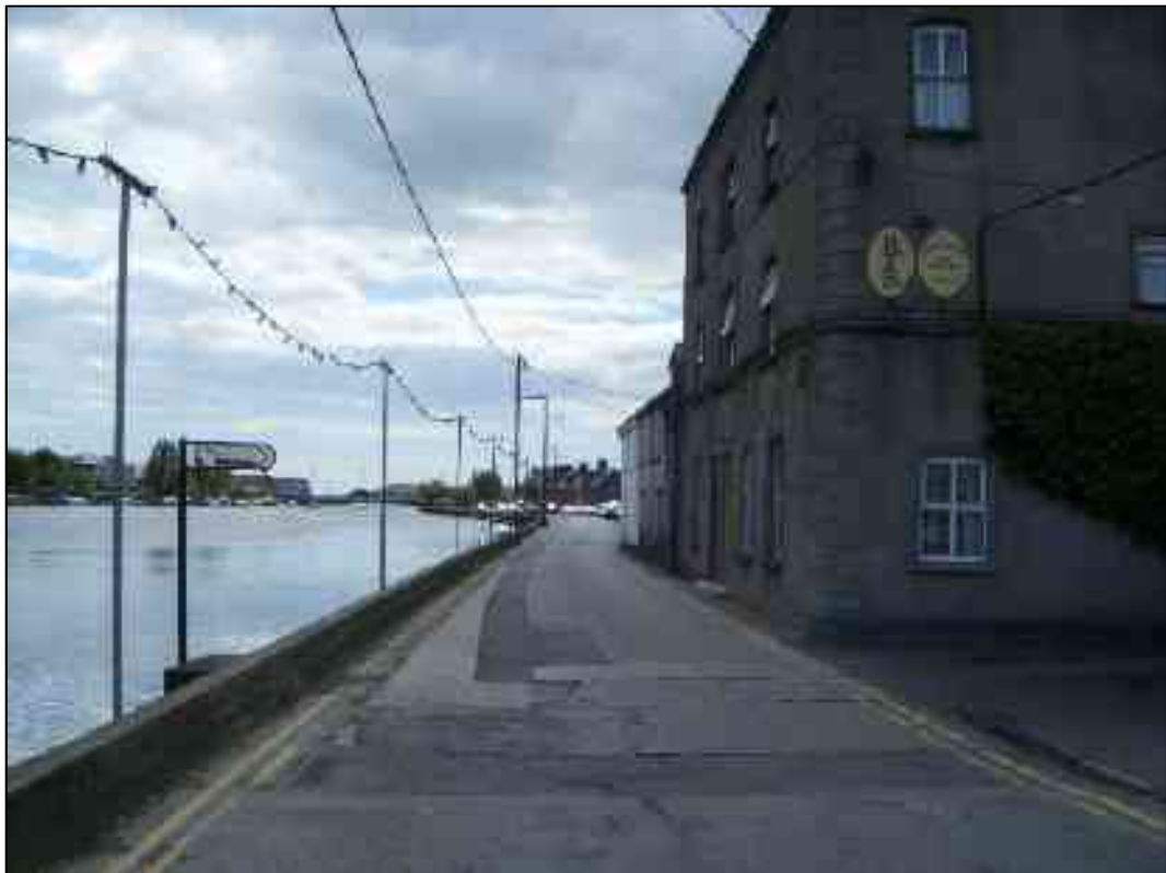
Figure 12 View of the west end of Section 2, looking east
