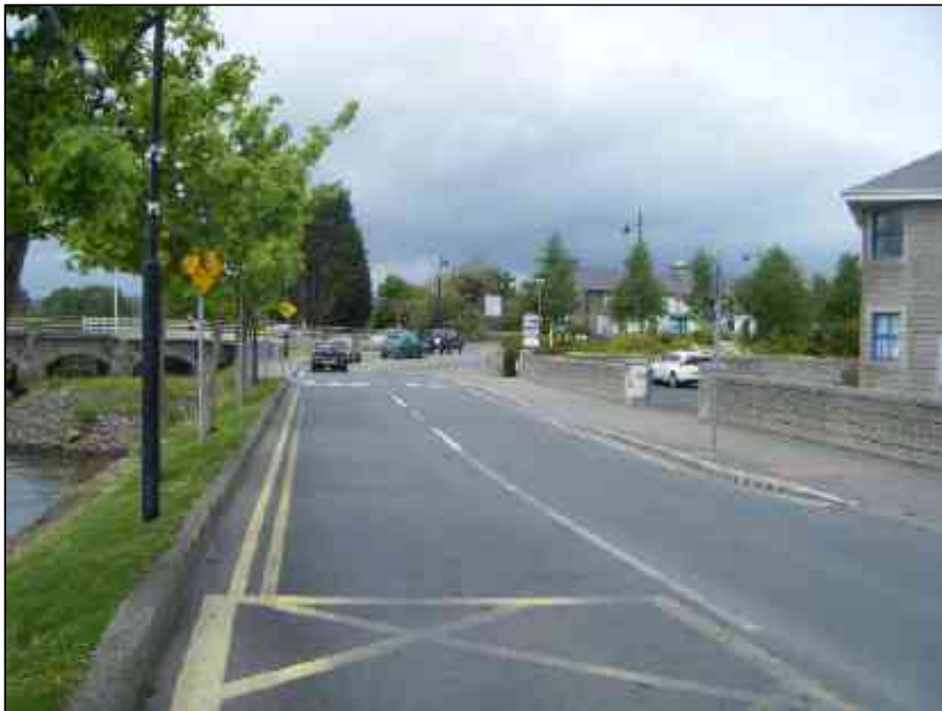
Figure 19 View of west end of Section 4, looking northwest
