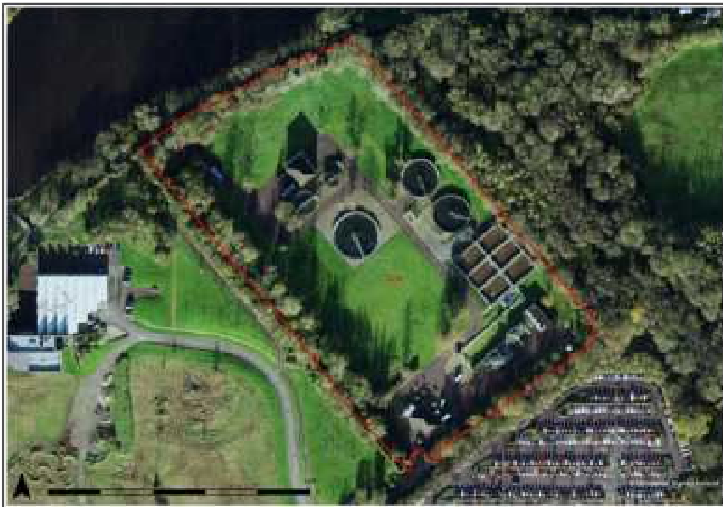
Figure 10-5: Aerial view, showing location of site.
