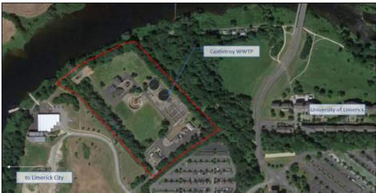
Figure 1: Location of Proposed Development (Source: Google Maps, annotation by J.B. Barry & Partners)
