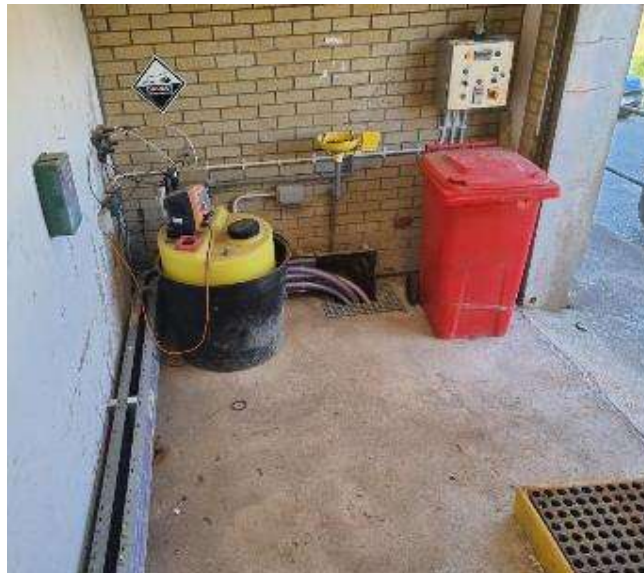
Figure 2: Disused Chlorine Room
