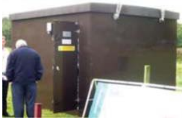
Figure 6 Typical orthophosphate dosing unit
