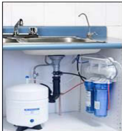
Typical POU Reverse Osmosis System. Photo: Rainfresh, Canada
