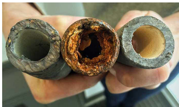
A lead pipe, a corroded pipe, and a pipe with protective orthophosphate coating. Photo: USEPA
