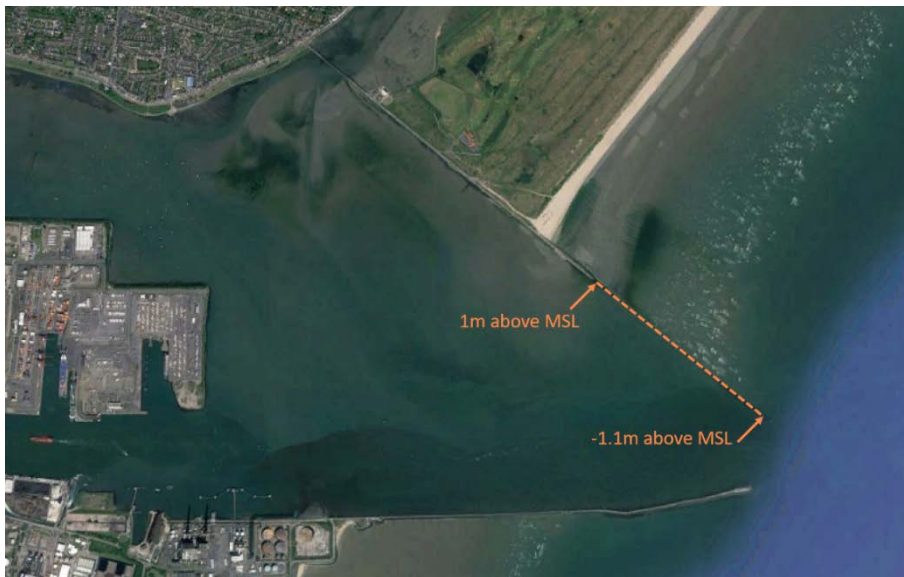
Figure 5.15 Aerial image of Dublin Harbour highlighting the semi-submerged section of the North Bull Wall (image Courtesy of Google Earth).
