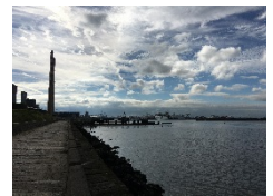
Ringsend WwTP outfall on the Lower Liffey Estuary at Poolbeg
