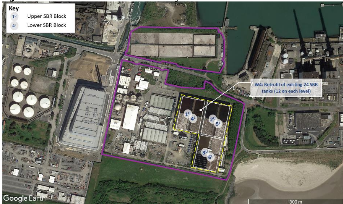
Figure 12: Location of SBR Tanks within the Ringsend WwTP site
