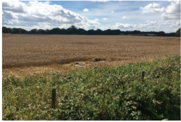
Example of valve chamber in a field at field boundary
