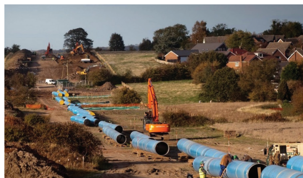
Pipeline corridor showing pipe before trenching and welding
