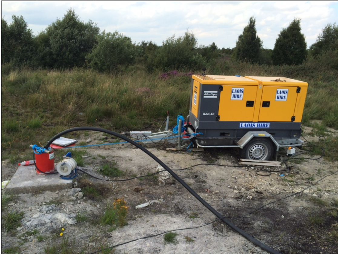
Plate A: Typical Pumping Test Setup (shown below at WH02)
